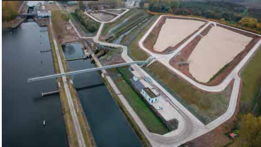
Treatment of dredged sediments, Vraimont - Belgium
