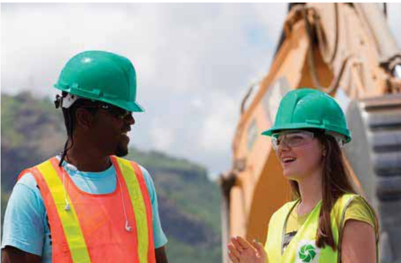
Capital dredging works Port Louis, Mauritius
