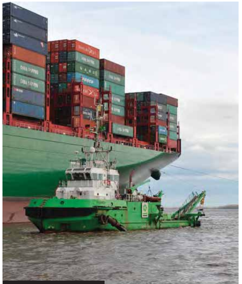
Water injection dredging on the Elbe for the salvage of the ‘CSCL Indian Ocean’, Germany
