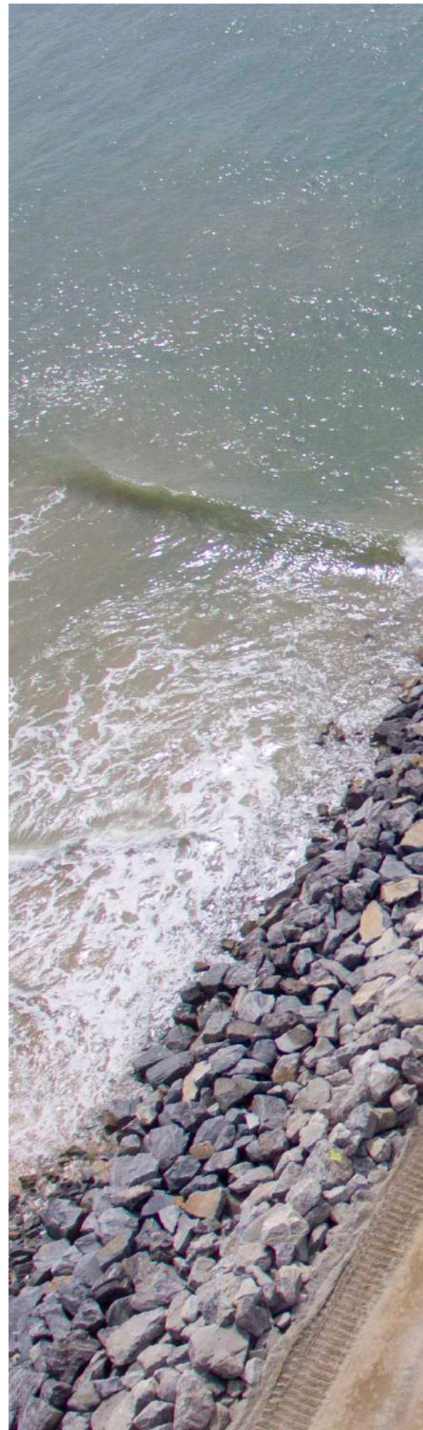
Cotonou - Benin Coastal protection works
