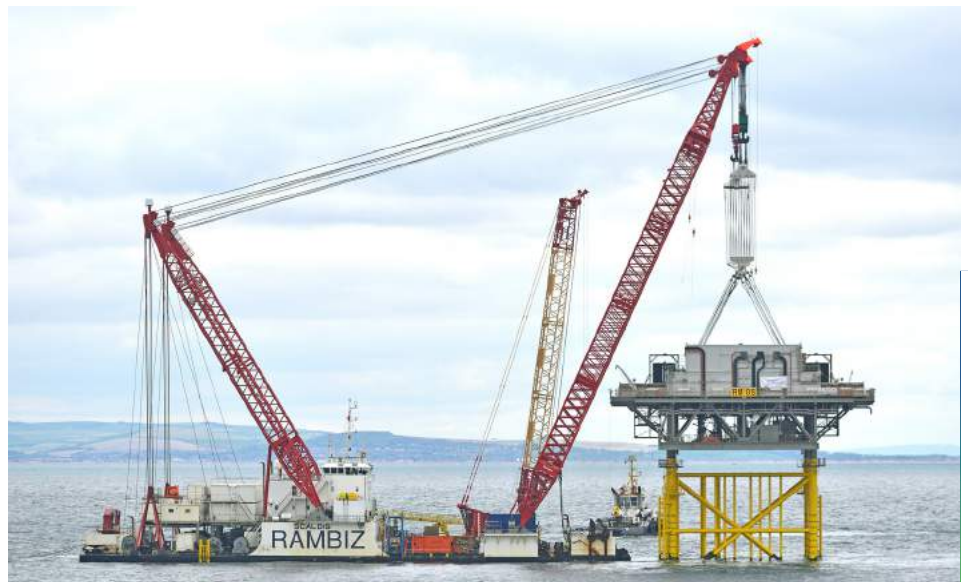
UK Transport and installation of the Rampion substation
