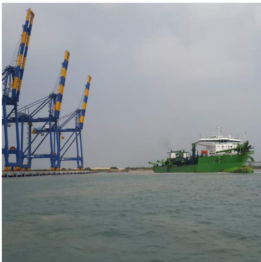
Kamarajar - India TSHD 'Congo River' at the Kamarajar port development project
