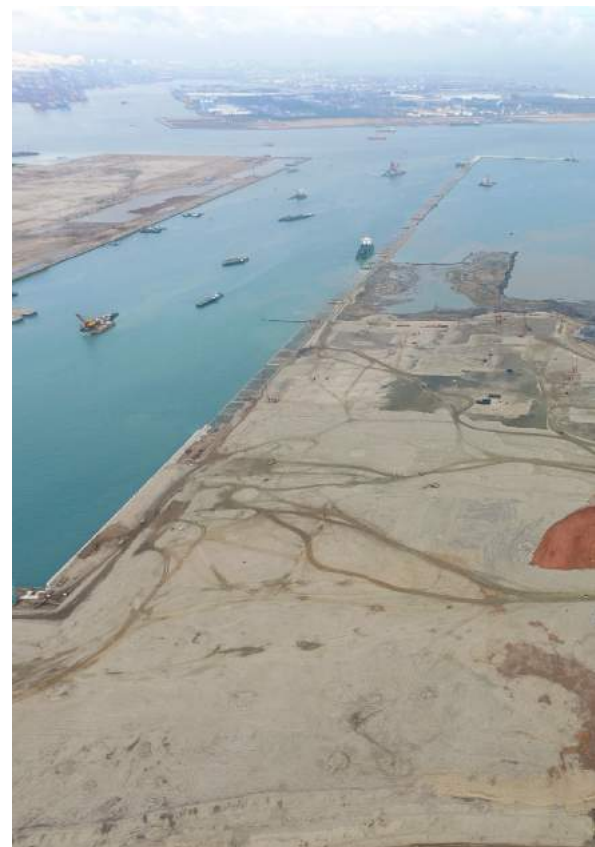
Singapore The TTP1 container terminal is clearly taking shape
