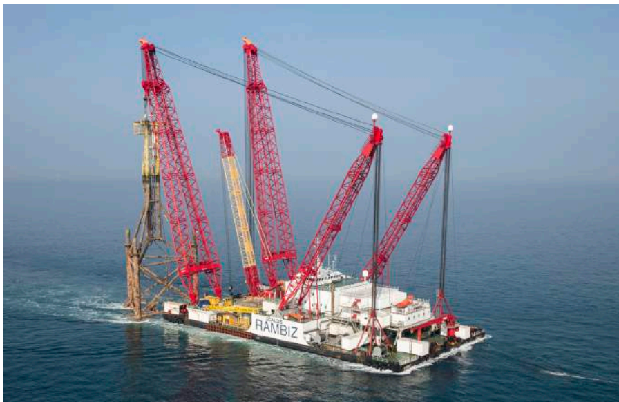
UK Horne & Wren decommissioning
