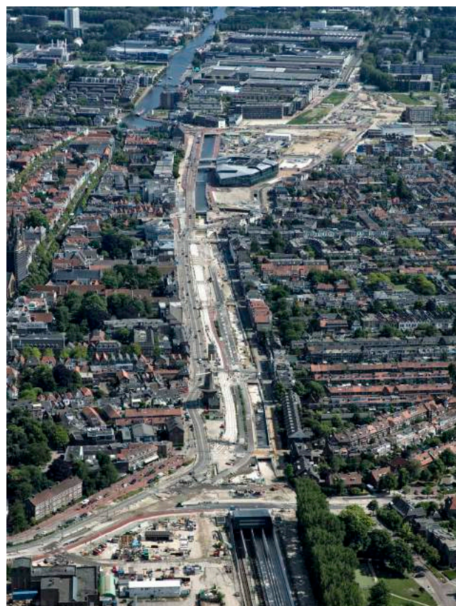
Delft - The Netherlands The Spoorzone Delft includes a 4-track rail tunnel
