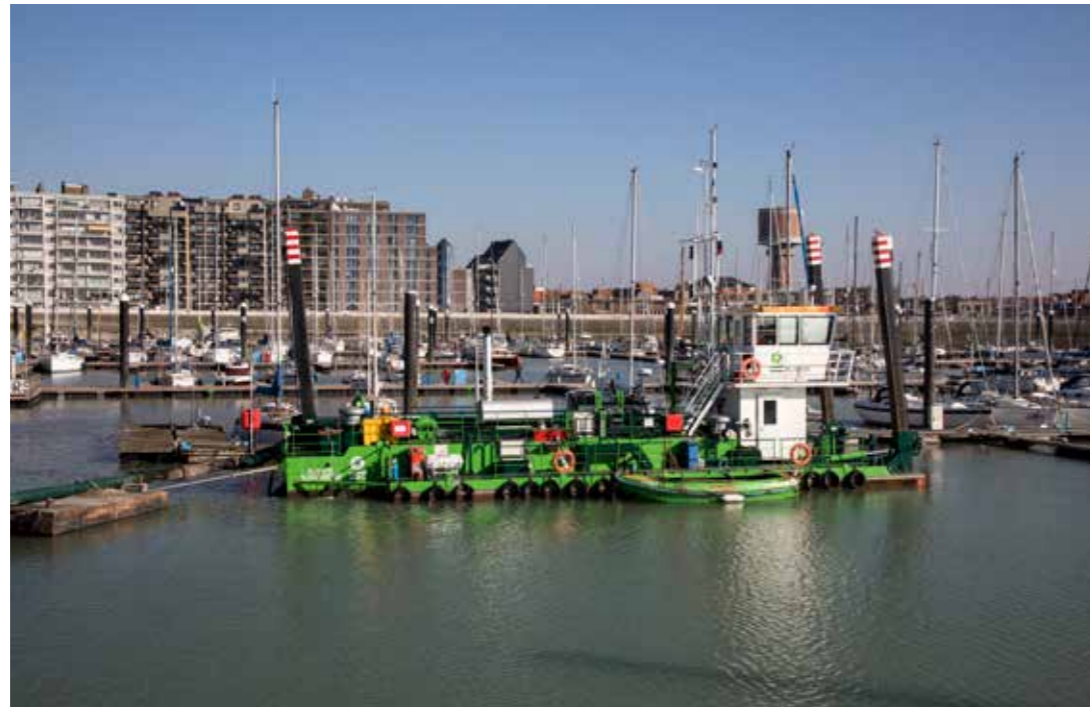
Electrical CSD 'Blanew'
